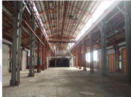
100 Series – Metal – looking south
