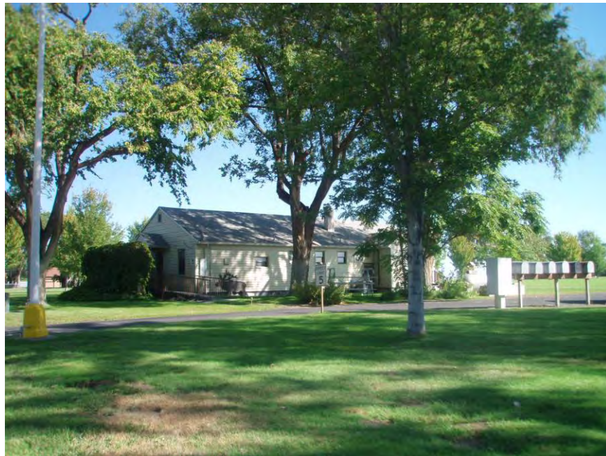
South and east elevation – entry with ramps
