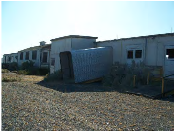
Ammo Operations Building (West bldg- North side)
