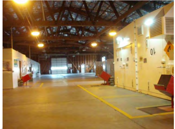
Building 31 East Half (West Half is Offices)
