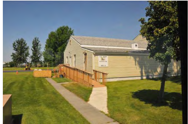
Building 33 South Entrance
