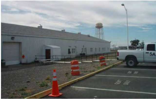
Building 31, North Side
