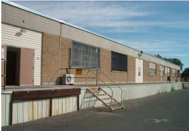
Building 11 Exterior looking Northeast
