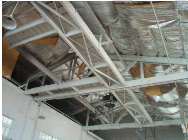
Roundhouse ceiling, North main bay
