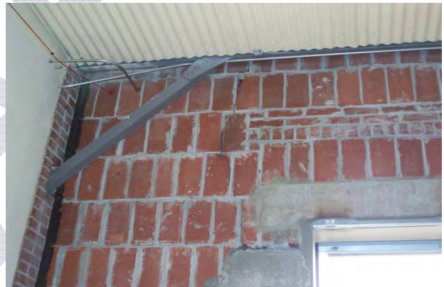
402 Building- Magazine Walls designed to blow
