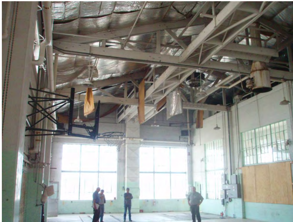
Roundhouse ceiling, north main bay looking southeast
