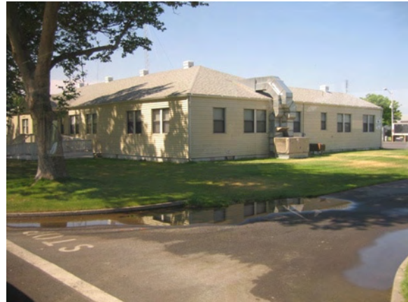
Operations Control Center looking Southwest
