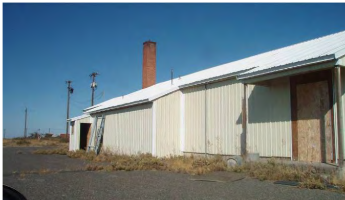
Ammo Operations Breakroom Building – North
