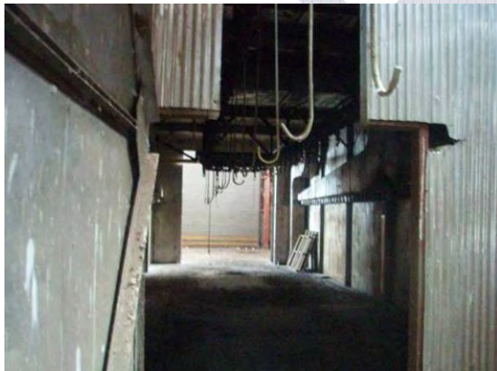
Munitions Paint Booth
