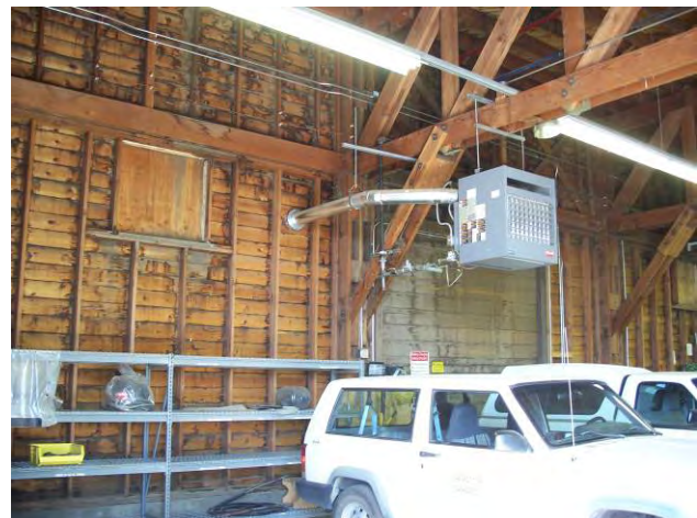
Re-used 200 Series Warehouse (New Unit Heater)
