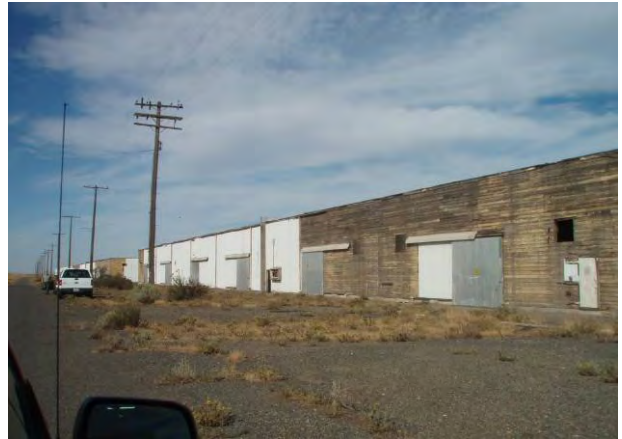
200 Series Warehouse, West Side
