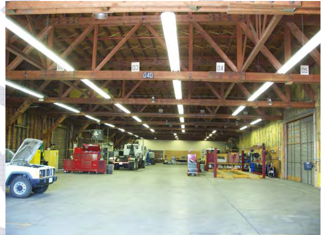
Re-used 200 Series Warehouse (New Lighting & Partition)
