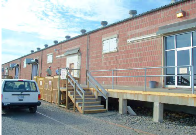
400 Series Buildings- Un-refurbished
