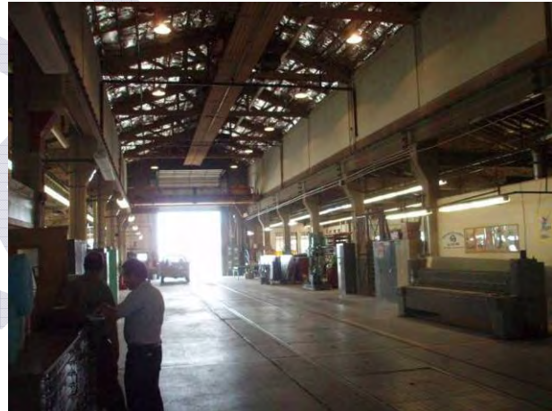
Maintenance Shop Building – Interior looking west
