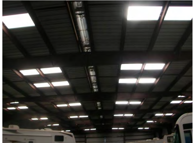
Bldg #450 (Skylighting only; automatic roof vents)
