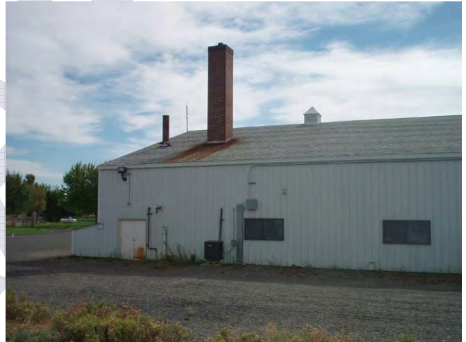
Building 31 N.E. Corner
