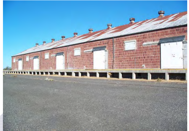
402 Building- Storage + Office -Refurbished
