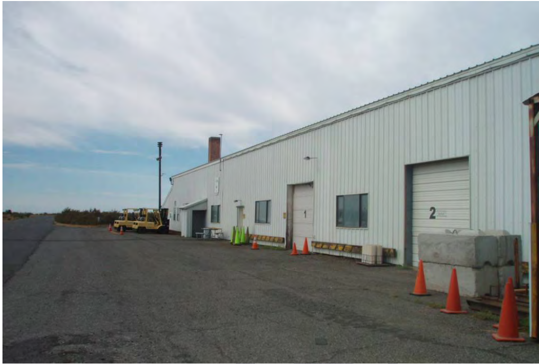
Dunnage – South Elevation
