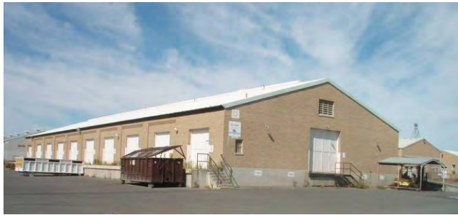
Building 17 Warehouse (Outside)
