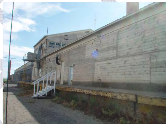
Concrete Warehouse (typ. of 3: built 1957-1960)
