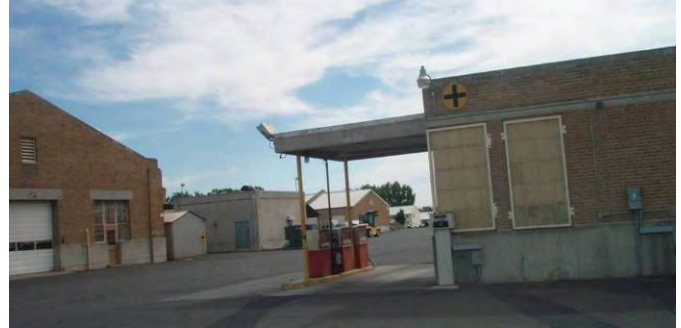
Gas Station looking south
