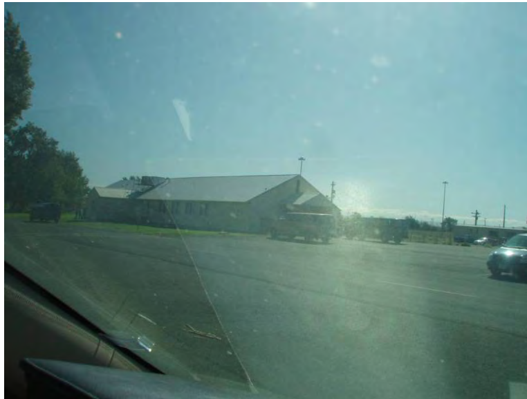
North and west elevations
