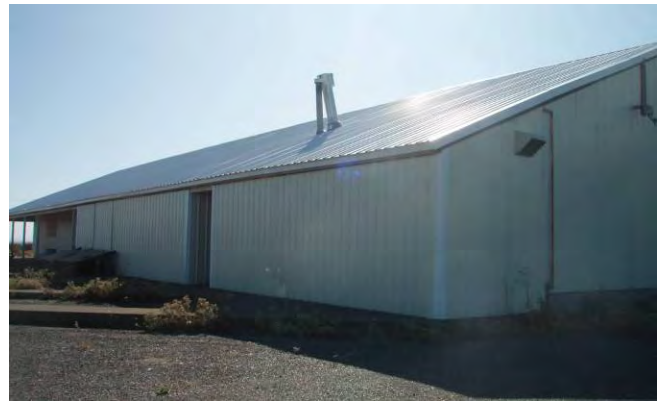
Ammo Operations Breakroom Building – South
