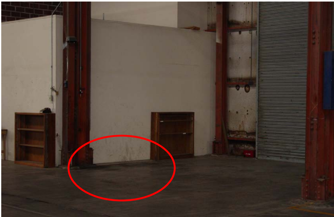
Figure 44. Building 115 – Former Location of Parts Washer (2004)
