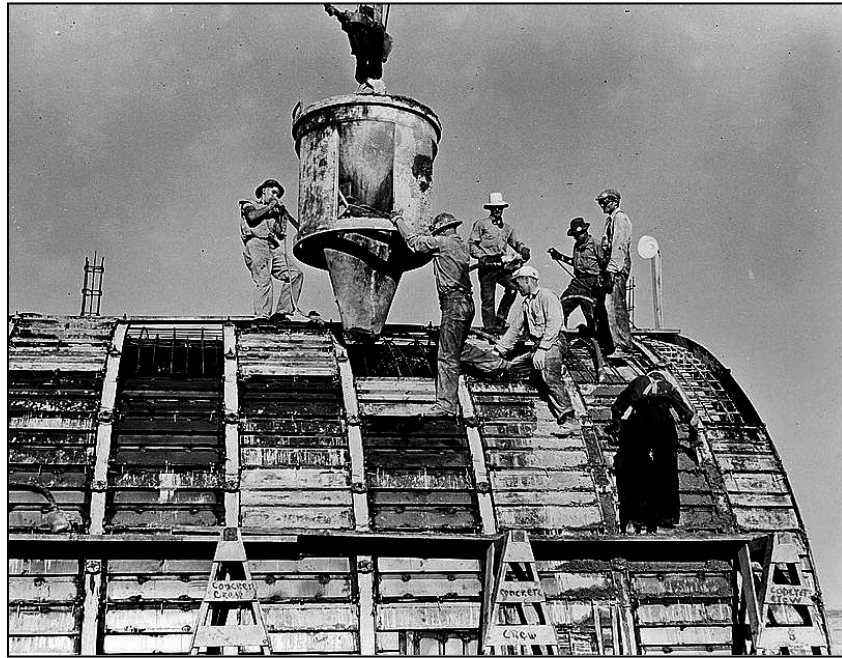
Figure 4. Construction of UMCD Igloos in 1941
