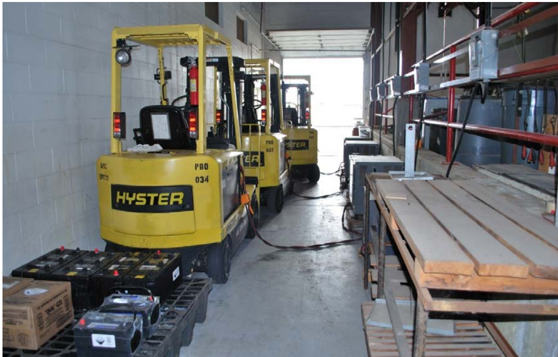
Figure 22. Bldg 27 – Battery Shop, East Wall, Looking South (March 2011)
