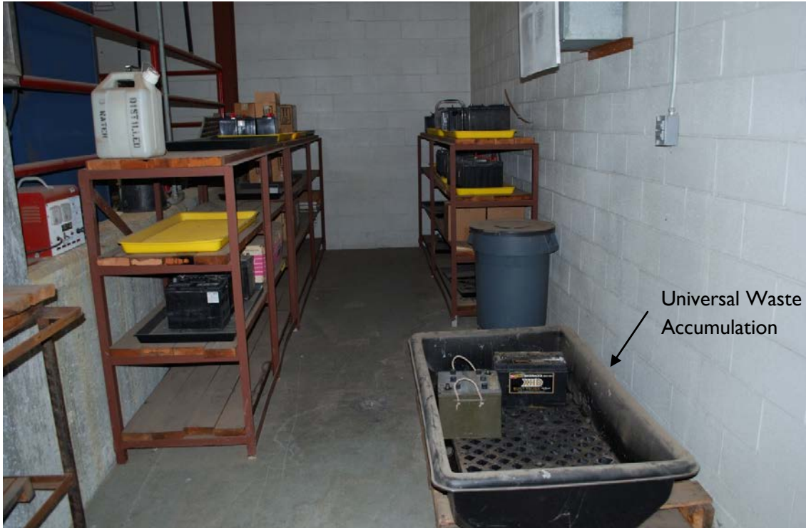
Figure 21. Bldg 27 – Battery Shop, East Wall, Looking North (March 2011)
