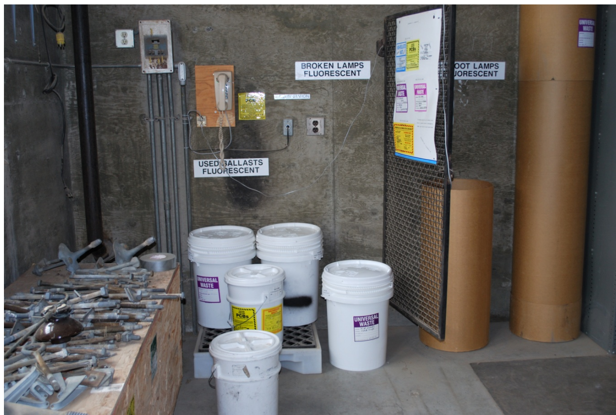
Figure 42. Building 14 Universal Waste SAA, Looking West (March 2011)
