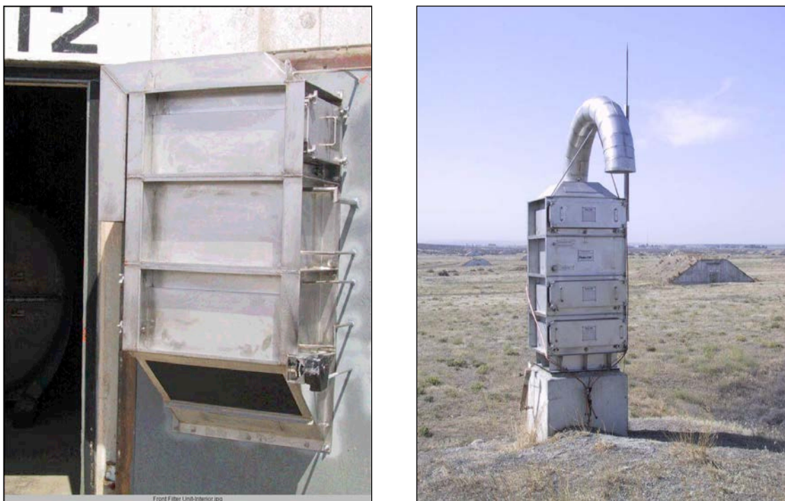
Figure 8. Front Passive Intake Filter and Rear Passive Exhaust Filters
