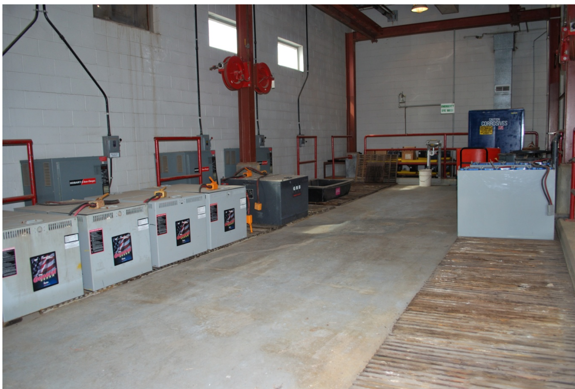
Figure 23. Bldg 27 – Battery Shop, Elevated Platform, Looking North (March 2011)
