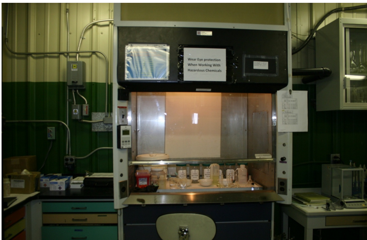
Figure 46. Building 656 SAA in Laboratory Fume Hood, Looking East (March 2011)
