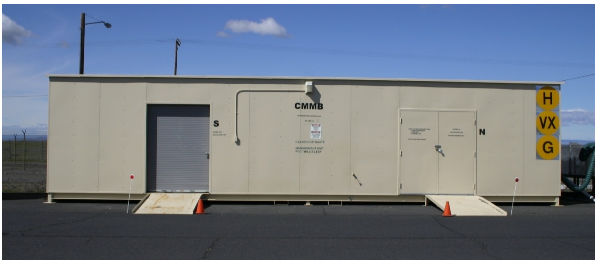
Figure 35. Containerize Material Monitoring Building, Looking Northwest (March 2011)
