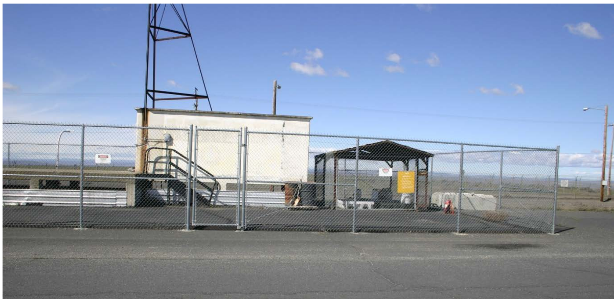
Figure 33. Pier 37 (Left) and Adjacent 90-Day Liquid Storage Area (Right), March 2011
