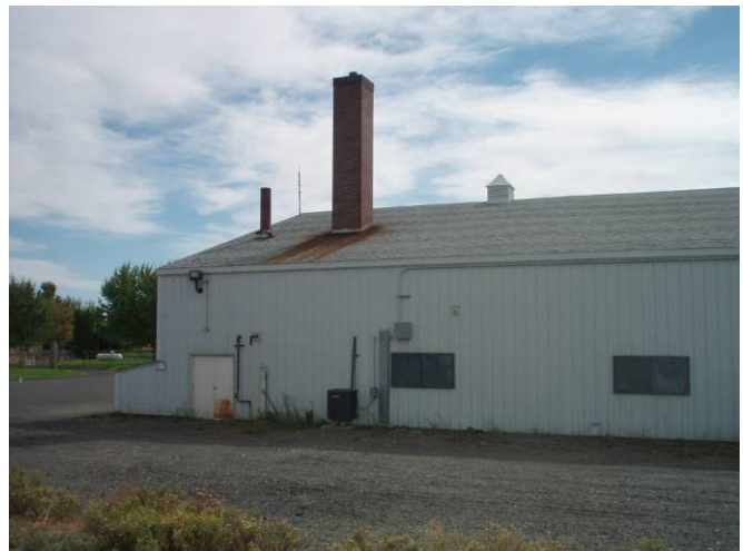
Building 31 N.E. Corner
