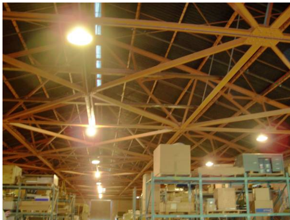
Building 17 Warehouse (Inside brightened photo)
