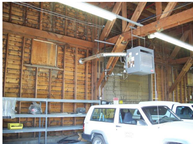
Re-used 200 Series Warehouse (New Unit Heater)
