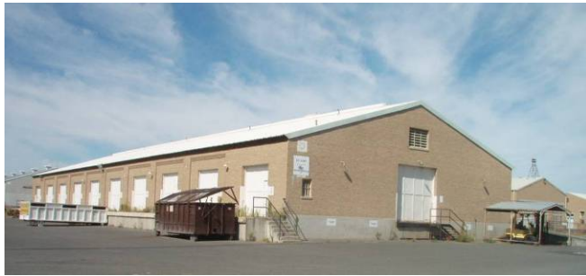
Building 17 Warehouse (Outside)
