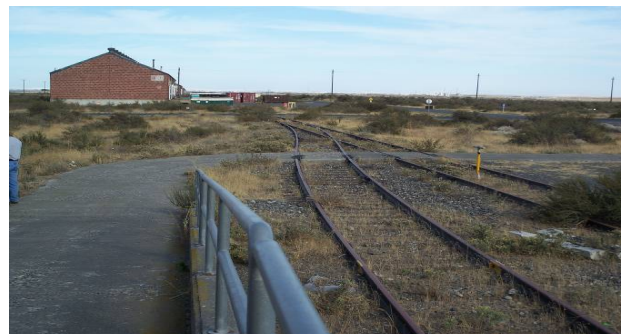
All 400 Buildings have looped rail access
