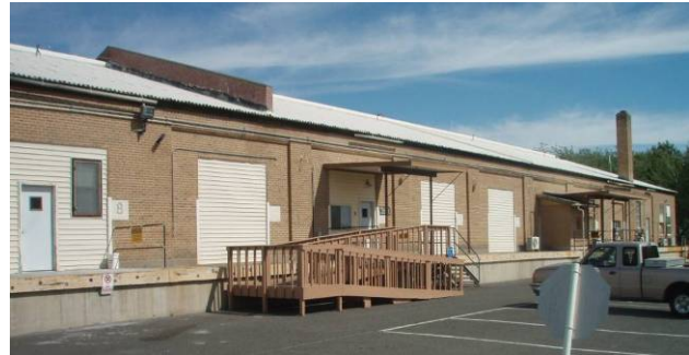
Building 18 Warehouse converted to office Similar to Building 11
