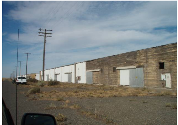
200 Series Warehouse, West Side
