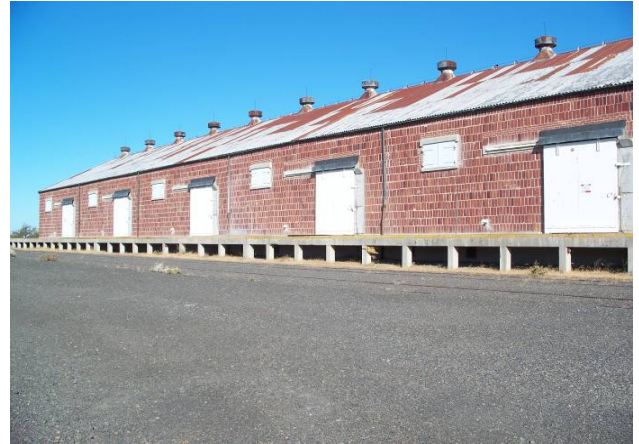
402 Building- Storage + Office -Refurbished
