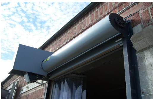
Building Motorized Roll-up Door (unused)
