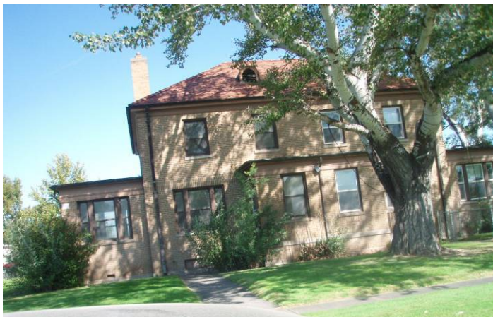
Duplex 16 from south
