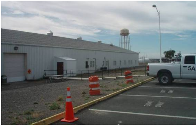
Building 31, North Side
