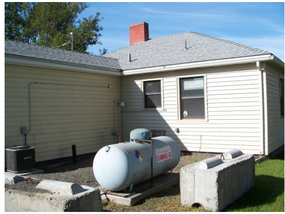
House #35 Northwest corner
