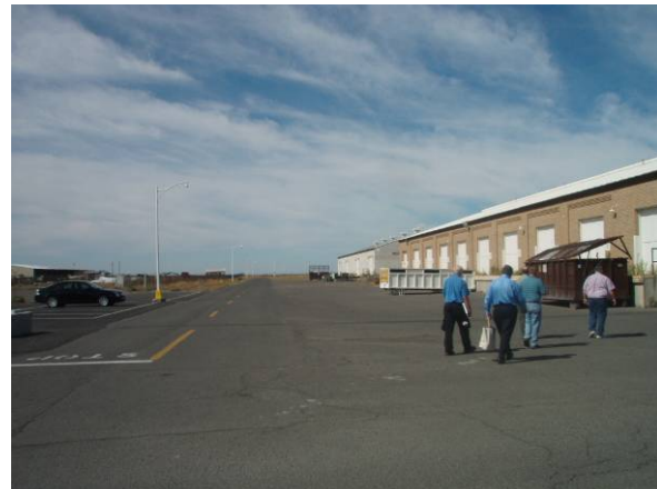
Building 19 Warehouse (background) Not toured- similar to Bldg 17)
