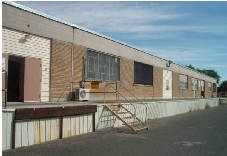
Building 11 Exterior looking Northeast
