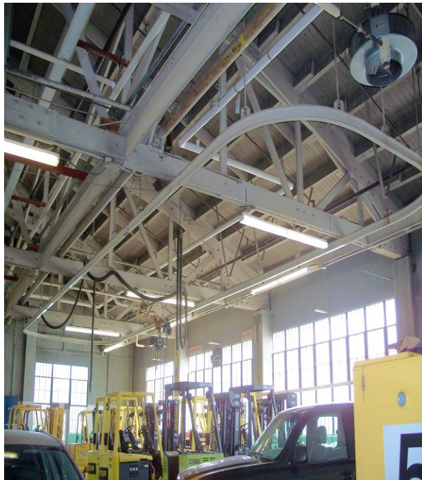
Monorail Hoists for Servicing Vehicles
