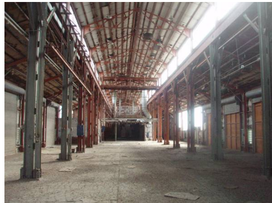
100 Series – Metal – looking south
