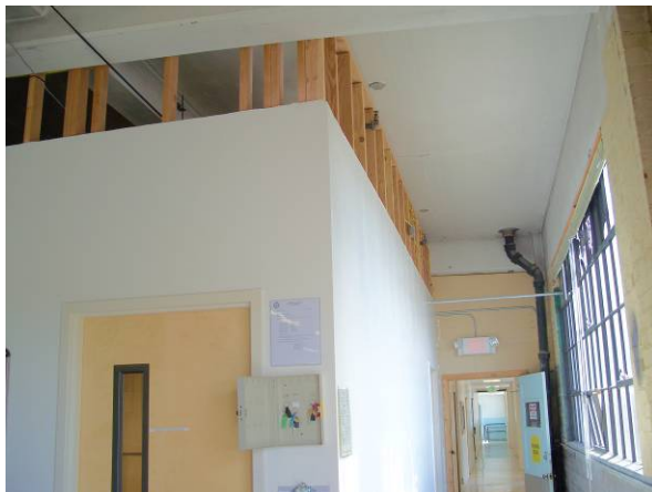
Building 11 Converted Warehouse to Offices Medical and Engineering Offices Looking East
