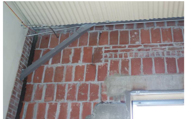
402 Building- Magazine Walls designed to blow outward
