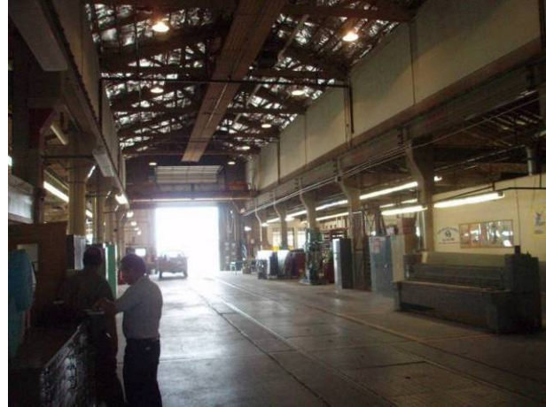
Maintenance Shop Building – Interior looking west
