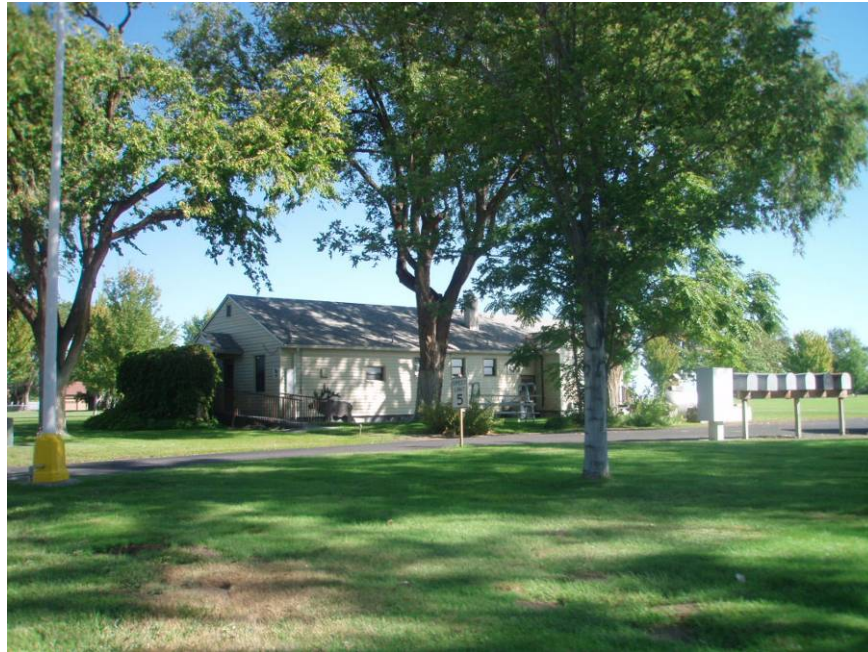
South and east elevation – entry with ramps
