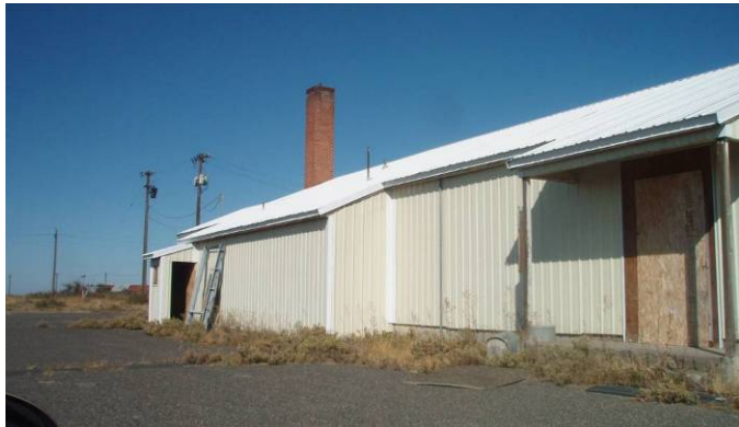
Ammo Operations Breakroom Building – South
