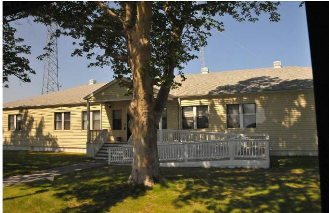
Operations Control Center looking West
