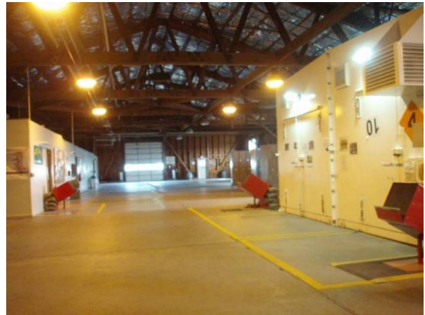
Building 31 East Half (West Half is Offices)
