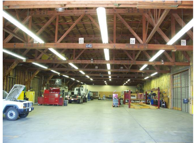
Re-used 200 Series Warehouse (New Lighting & Partition)
