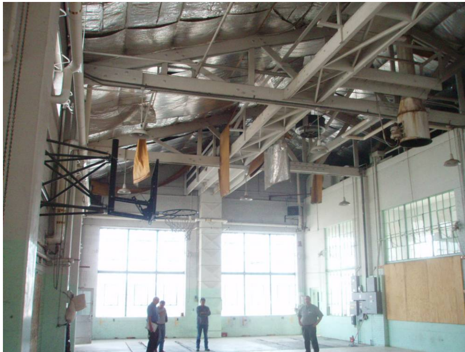
Roundhouse ceiling, north main bay looking southeast
