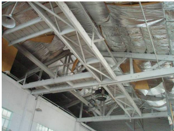
Roundhouse ceiling, North main bay
