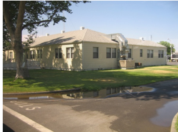
Operations Control Center looking Southwest
