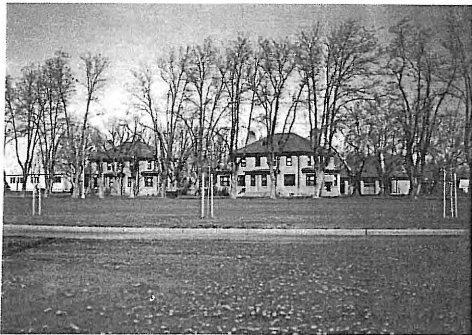
Original brick residences along Circle Drive (Bldgs. 15, 16, 70)
